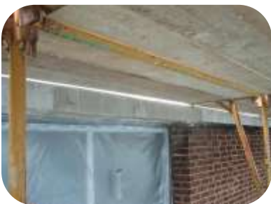
Damaged lintel rebuilt with 571 Concrete Repair LW
