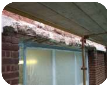
Damaged lintel rebuilt with 571 Concrete Repair LW
