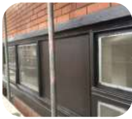
Lintels rebuilt with 571 Concrete Repair LW
