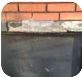
Lintels rebuilt with 571 Concrete Repair LW
