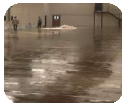
Concrete surface on a chemical containment area was mechanically abraded and sealed with Resichem 503 SPEP prior to being over coated with Resichem 501 CRSG
