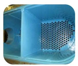
Heat exchangers are prone to bimetallic corrosion on tube sheets, end covers and water boxes.
