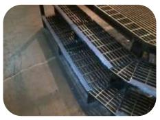
Stair nosings in an oil refinery could only be manually abraded. The metal surface had ingrained oils and grease and were wiped down with solvent.
