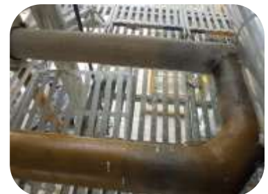
Cold water lines at operating at 5°C. The ambient temperature was measured at 32°C on average with humidity at 85%. 560 Thermal Barrier XF was applied at 8mm around the pipework to eradicate condensation build up
