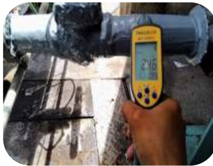
Cold water line at a chemical plant operating at 2-4°C. The ambient temperature was measured at 32°C on average with humidity at 65-85%. 560 Thermal Barrier XF was applied at 8mm around the pipework to eradicate condensation build up
