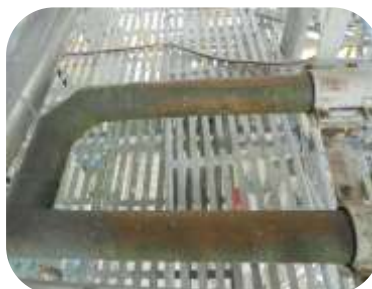
Cold water lines at operating at 5°C. The ambient temperature was measured at 32°C on average with humidity at 85%. 560 Thermal Barrier XF was applied at 8mm around the pipework to eradicate condensation build up
