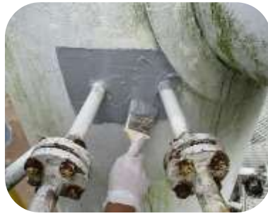
External tank surface prone to condensation and mould growth was abraded and coated with 4mm of 560 Thermal Barrier XF
