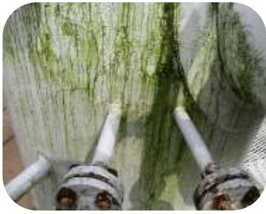
External tank surface prone to condensation and mould growth was abraded and coated with 4mm of 560 Thermal Barrier XF
