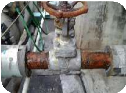
Cold water line at a chemical plant operating at 2-4°C. The ambient temperature was measured at 32°C on average with humidity at 65-85%. 560 Thermal Barrier XF was applied at 8mm around the pipework to eradicate condensation build up
