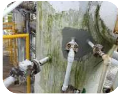
External tank surface prone to condensation and mould growth was abraded and coated with 4mm of 560 Thermal Barrier XF
