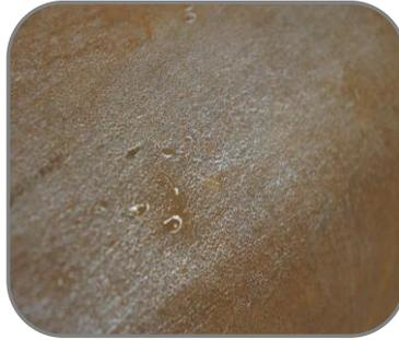
All loose materials and corrosion must be removed
