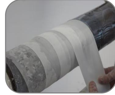
Then wrap the glass tape along the length of the pipe ensuring you overlap the glass tape by 50%
