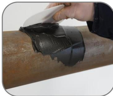
Apply the mixed material to the abraded pipe surface
