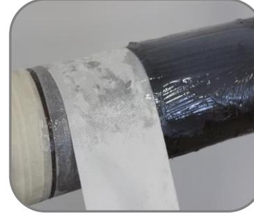
Wrap the glass tape around the pipe 3 times to create an anchor point
