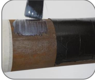
Apply the mixed material at 1mm WFT using a brush
