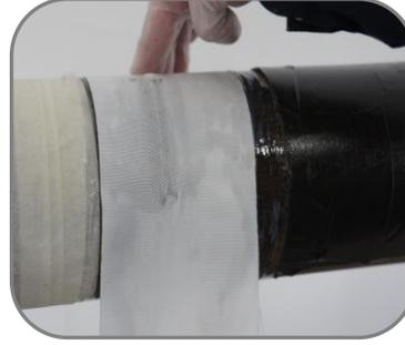
While the resin is still wet begin to wrap glass tape around the pipe
