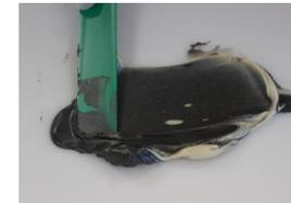
Apply to the pipe surface using the applicator tool
