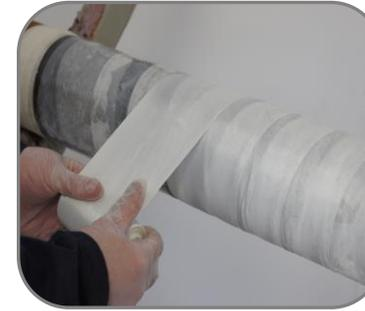
After the 2<sup>nd</sup> wrap of glass tape has been terminated. Apply 301 Epoxy Resin & Hardener at 500 microns WFT and repeat the glass tape wrapping process for a 3<sup>rd</sup> and final time
