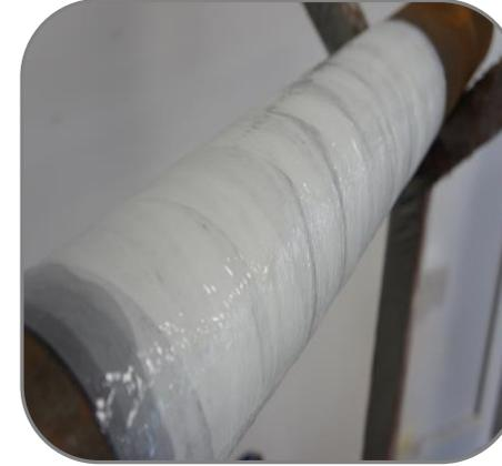
The completed system will range from 2-5mm dry film thickness depending on how much 302 Epoxy Repair Cement has been applied.
